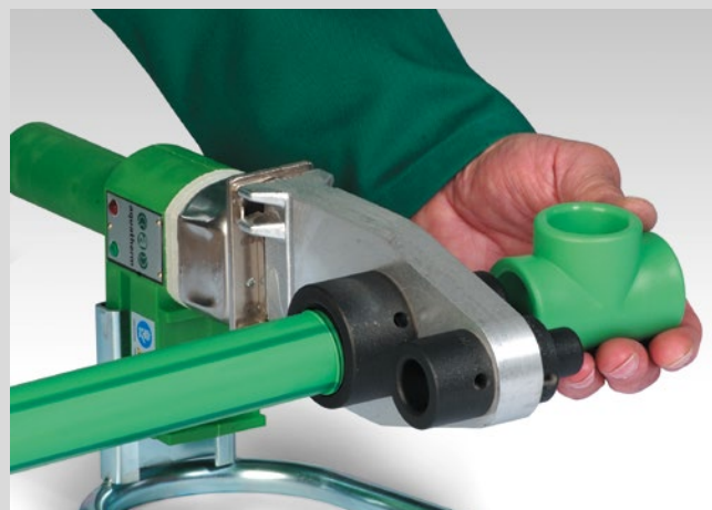
Heating-up of pipe and fitting
