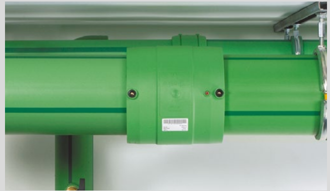
Push the second pipe – also peeled and cleaned – into the socket
