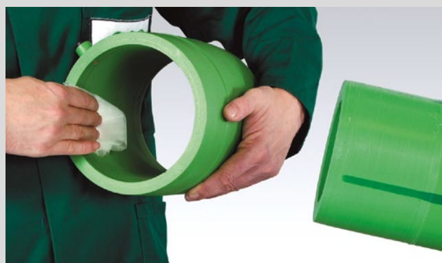
Clean the electrofusion socket's inner surface with a lint-free cloth or paper. Remove moisture that may occur immediately before the welding process again.
